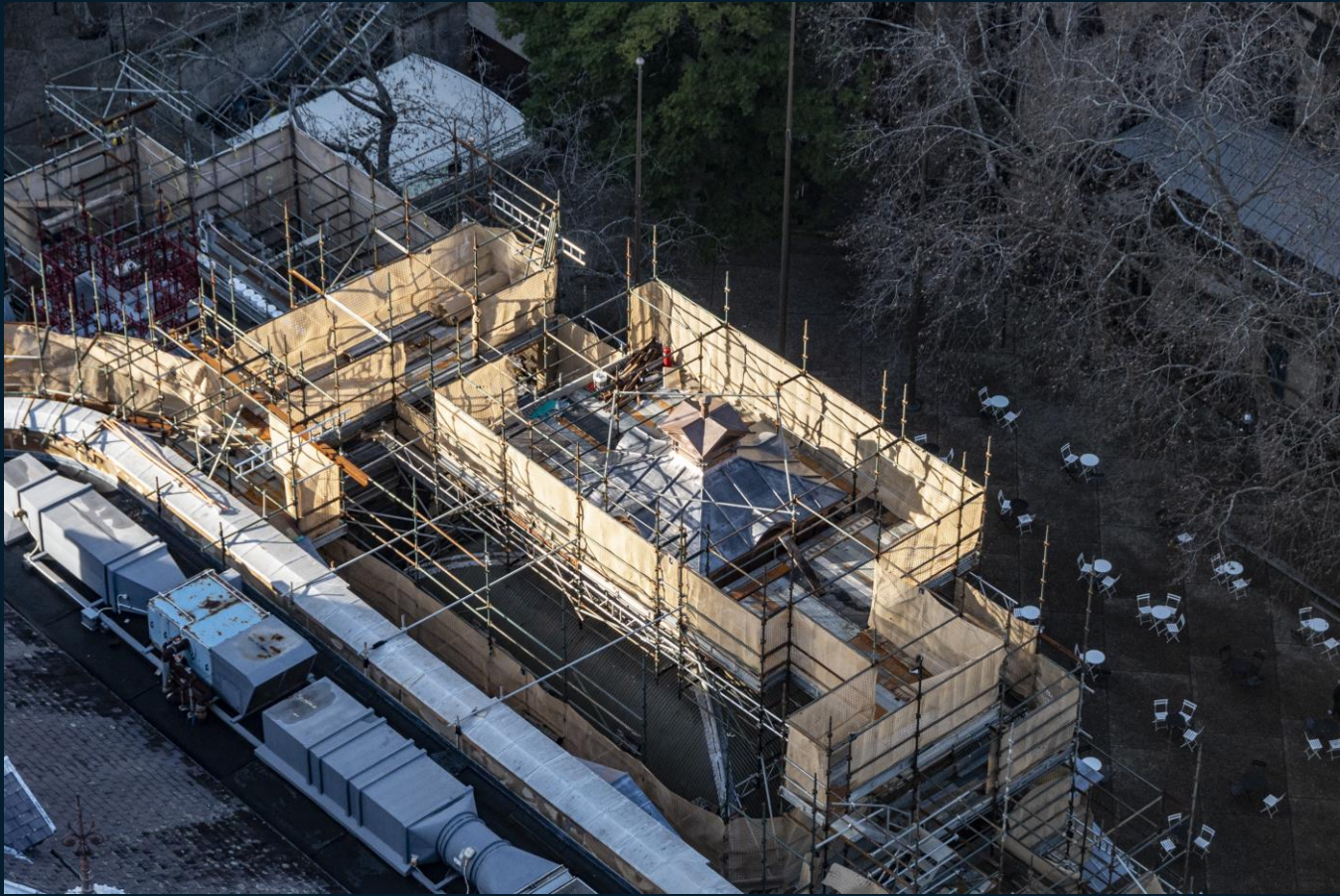
SYDNEY TOWN HALL EXTERNAL WORKS - STAGE 3
