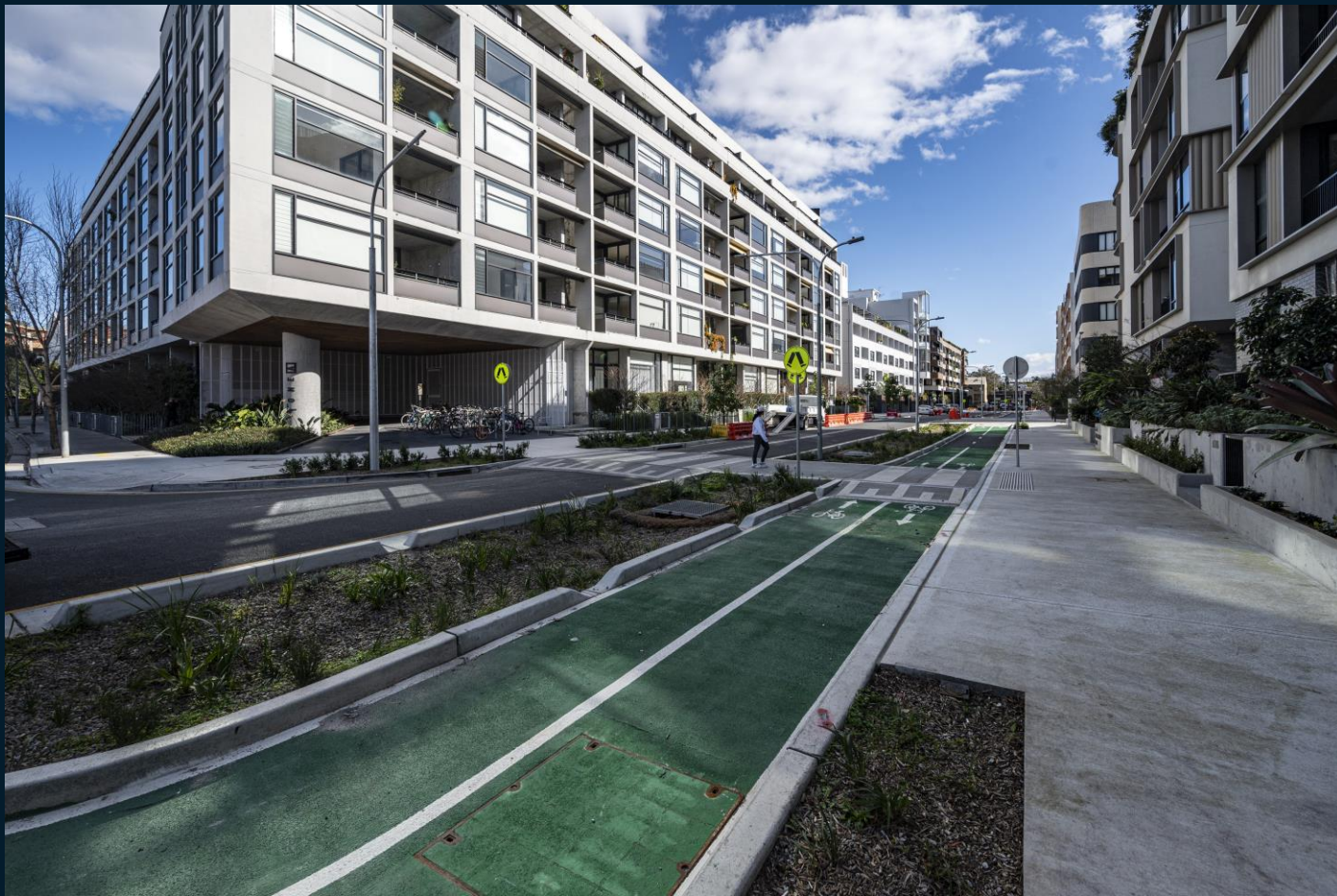
MACDONALD ST WIDENING WORKS, ASHMORE/ERSKINEVILLE
